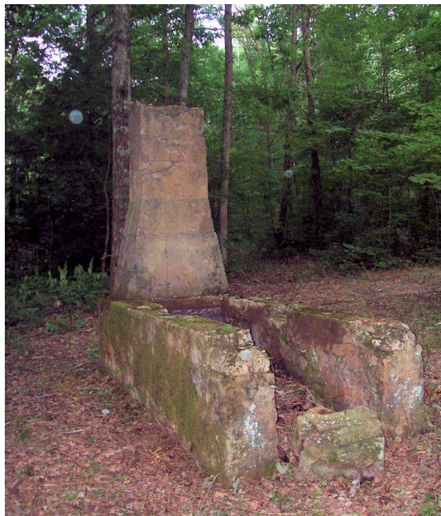
Below: another view of the boiler
