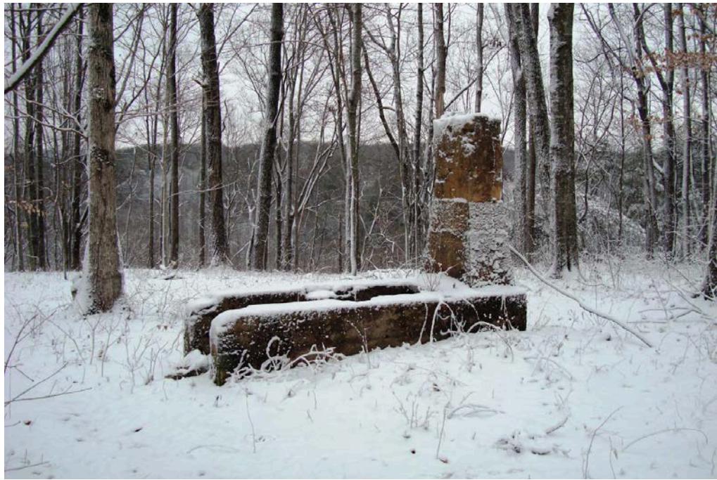
Above: the boiler setup showing how close to the bluff the operation was located.
