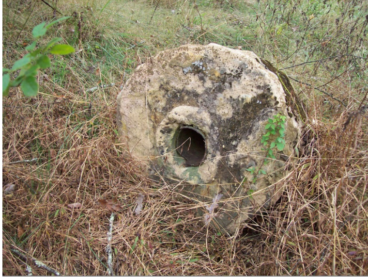
The broken casing of the old well surrounded by concrete – the well itself is still present but safely covered.
