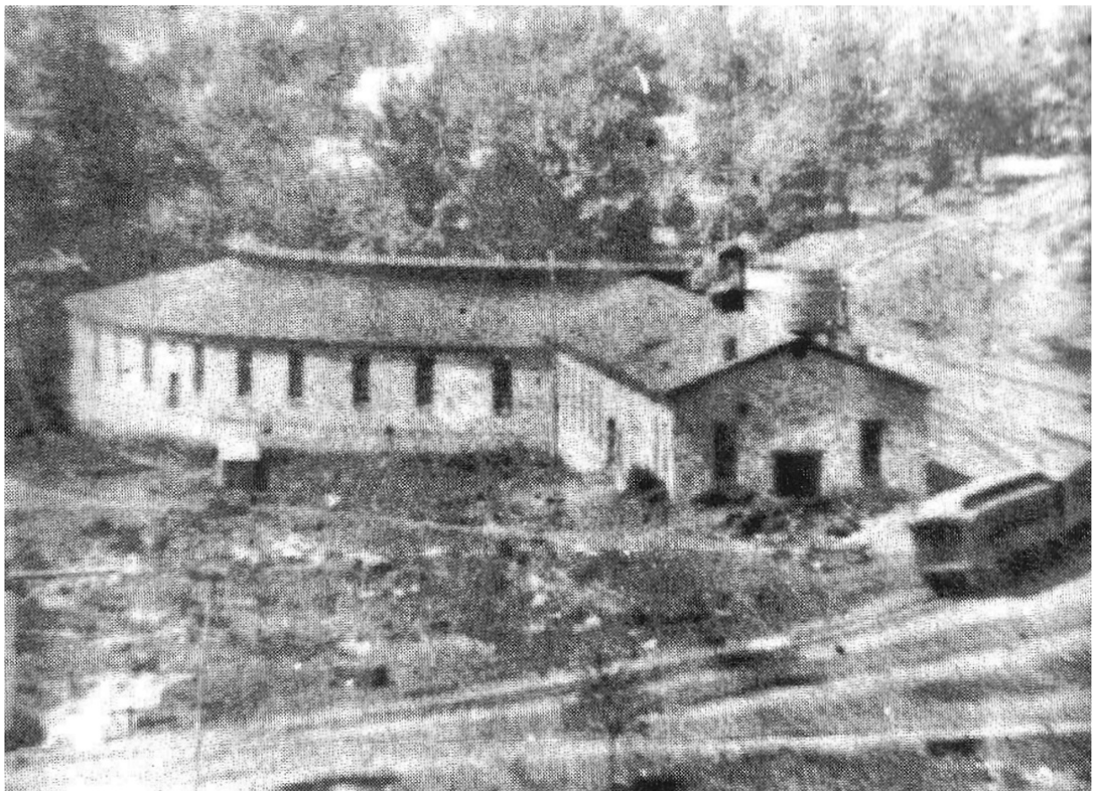
Round House in Tracy City (photo taken 1889); Wm. H. Bolton's engine and all others were turned around here for the next assignment. The railroad leaving town for Cowan can be seen in upper right-hand corner of photo.
