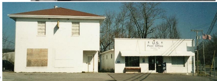
Bottom right: Pelham Post office & lodge building
