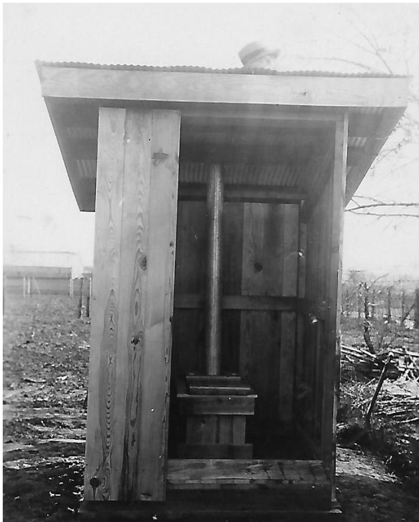
Sanitary pit privie under construction
