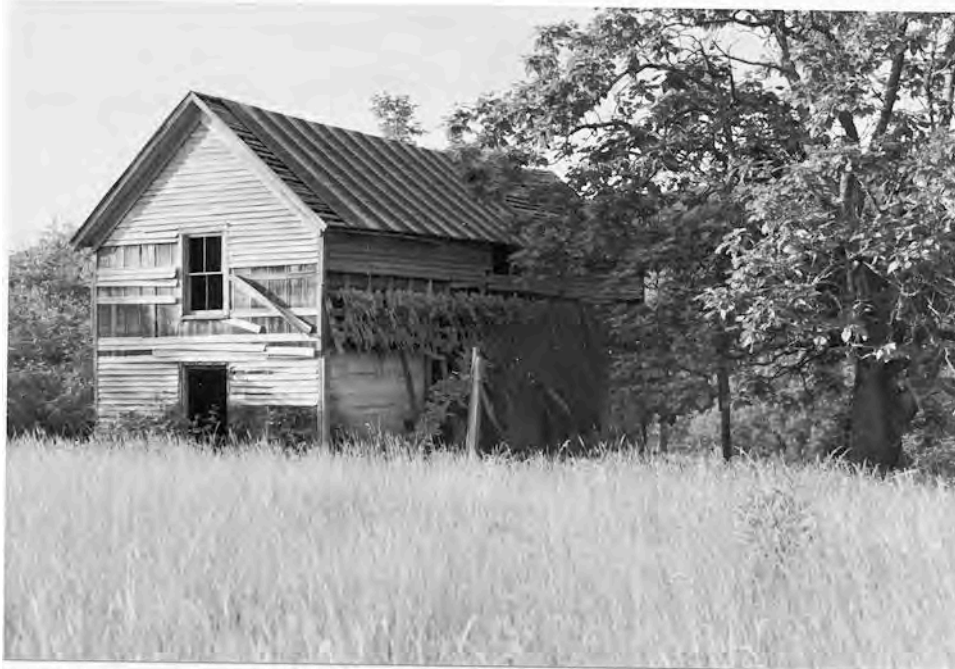
J. H. H. Boyd House Built ca 1897
