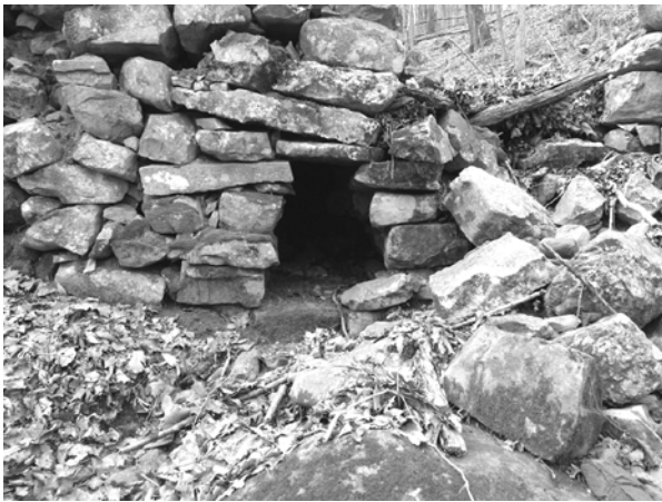
A culvert on Payne's Turnpike
