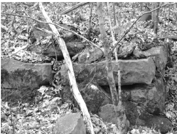
A corner foundation of the Toll House
