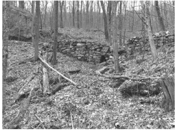
A retainer wall on Payne's Turnpike
