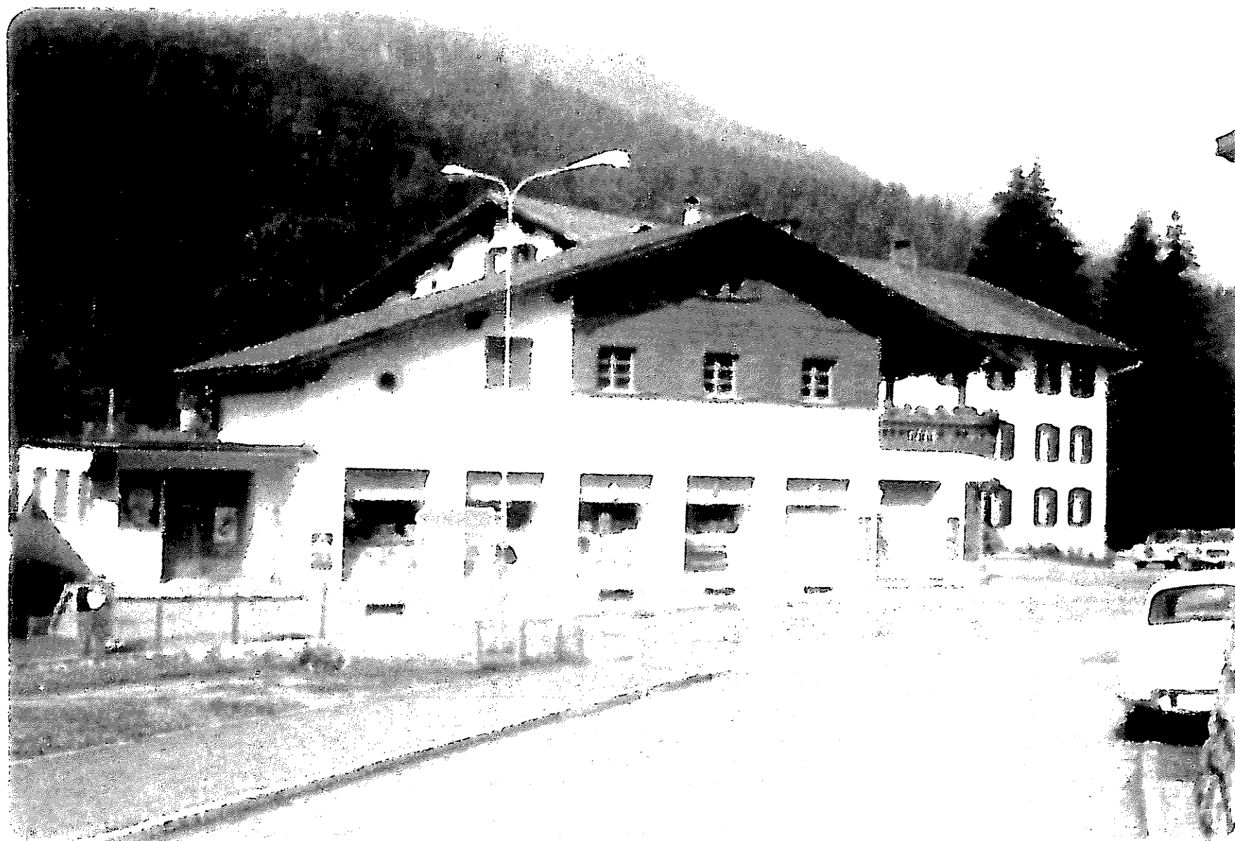
Marugg Ancestral Home in Klosters, Commercial Shops in Front of Main Living Quarters and Guest Rooms
