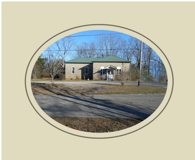
Hobbs Hill School/Community Center in 2017 (without metal awning on the right end of the building--jackie)
