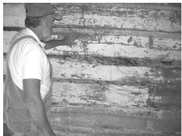
Grady Ward Partin, a true mountain man, inspects the "chinking and dobbing" between the logs.
