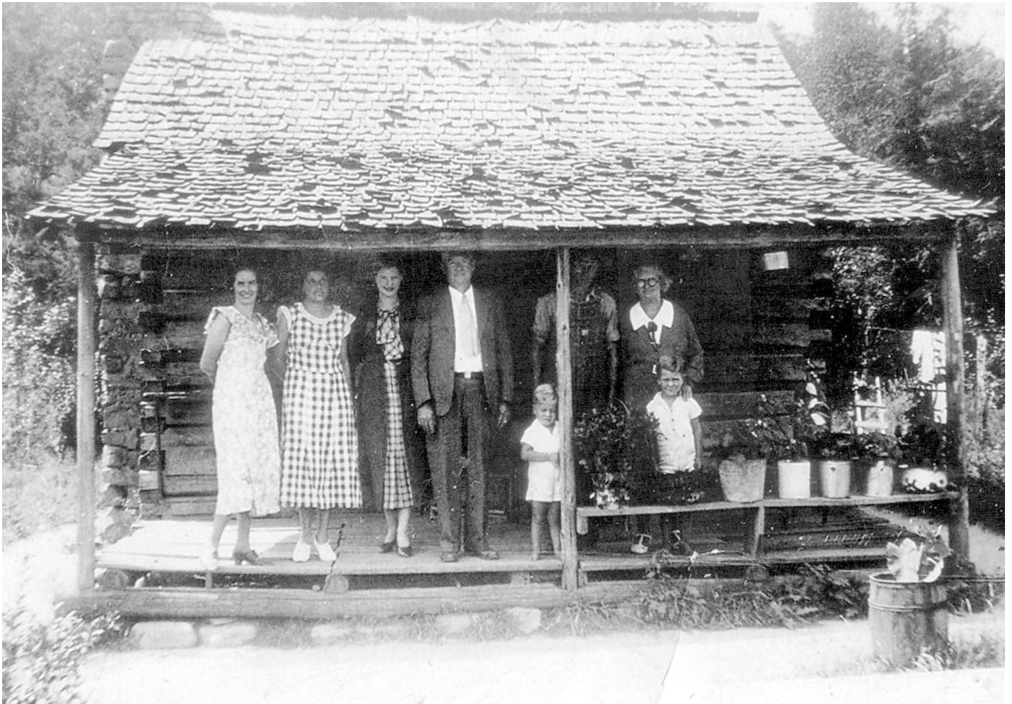
Ernest Rubley Home – “The House by the Side of the Road”
