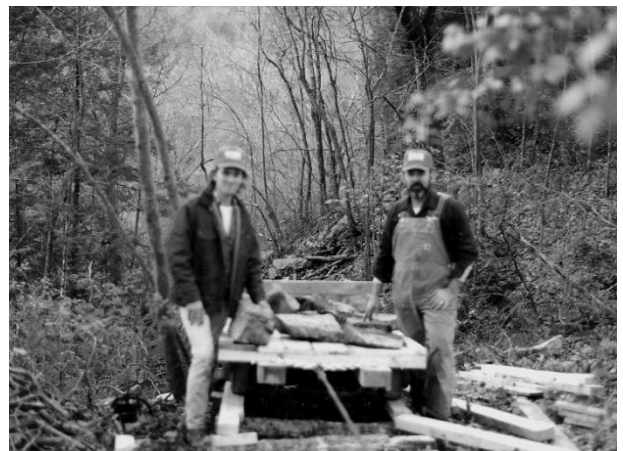
Left: Curt Partin and his father, Grady Ward Partin with their first load of rock brought out on their tramway
