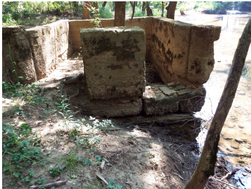
Bell's Mill sluice area with the water entrance and exit clearly seen
