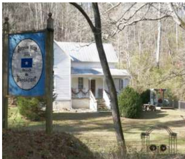
After construction of Bonnie Blue
