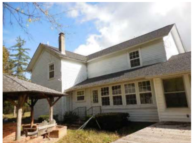
Figure 5. Rear elevation of house showing enclosed porch.
