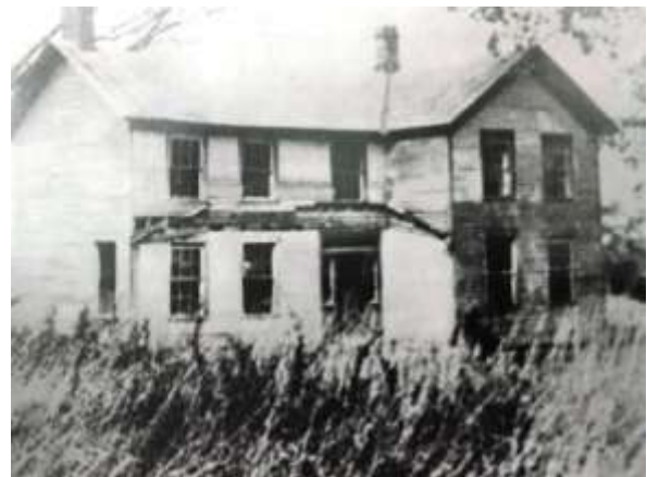
Clifford McClain House prior to remodeling
