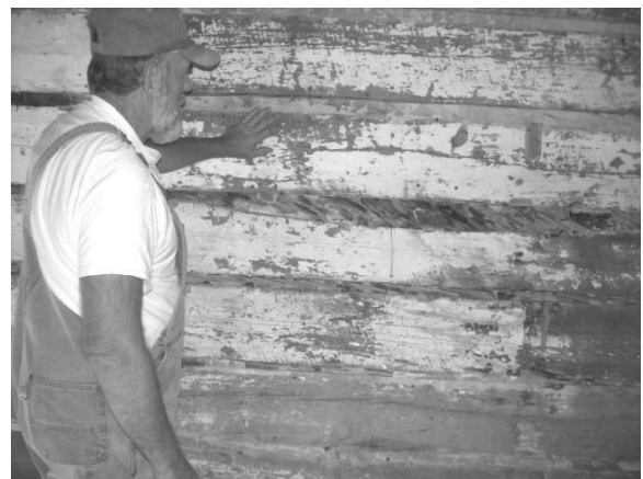
Grady Ward Partin, a true mountain man, inspects the "chinking and dobbling" between the logs.
